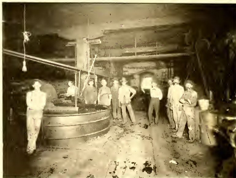
INTERIOR VIEW OF BEATER ROOM
